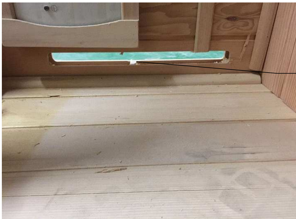
Photo 6 - Inlet ventilation
